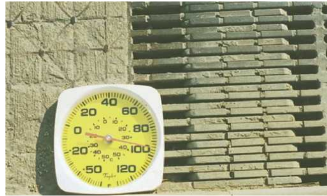
Figure 5.8 Expansion joints allow for the thermal expansion of bridges and other elevated roadways. Each end of a section of the roadway is connected to a metal “comb.” The teeth of the two combs fit together and can move back and forth as the lengths of the sections change. For comparison, the thermometer is 30 centimeters (1 foot) wide.
