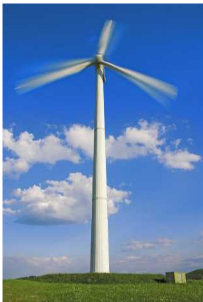
Figure 3.26 This wind generator converts kinetic energy of the wind into electrical energy plus some internal energy because of friction.
