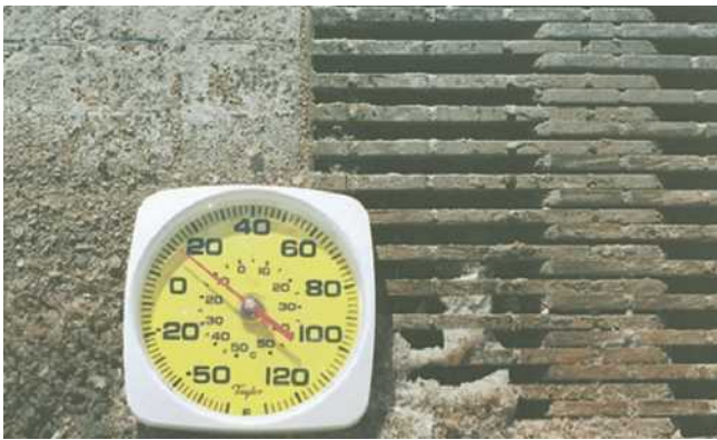
Figure 5.8 Expansion joints allow for the thermal expansion of bridges and other elevated roadways. Each end of a section of the roadway is connected to a metal “comb.” The teeth of the two combs fit together and can move back and forth as the lengths of the sections change. For comparison, the thermometer is 30 centimeters (1 foot) wide.
