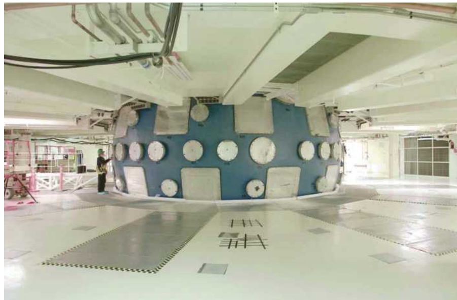
Figure 11.28 The 10-meter-diameter target chamber (blue) during construction of the National Ignition Facility. An assembly of 192 high-powered laser beams will converge on a fuel capsule at the center of the chamber.
